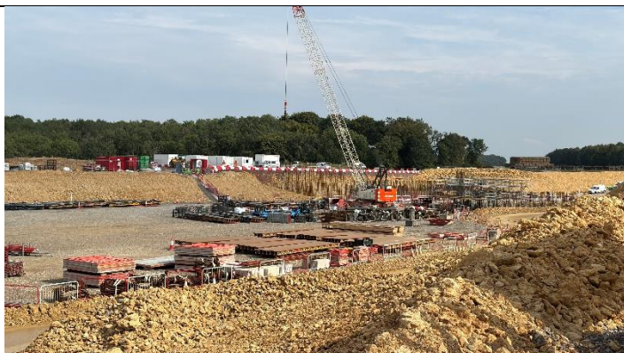
Construction of the 'Nature Bridge'
