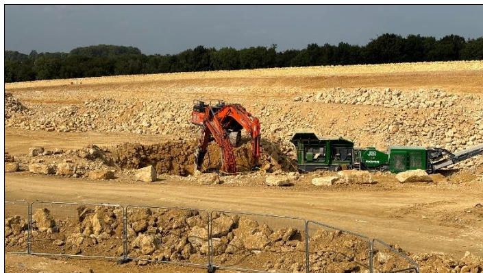
Excavators and crushing machine at Shab Hill
